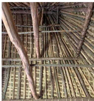
Figure 4-9: Use of bamboo for roof support trusses and thatching support bracing in bure
