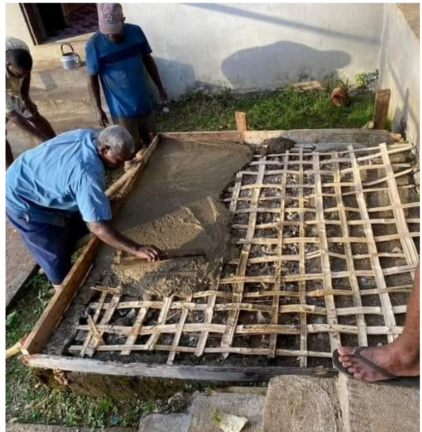
Figure 6-5: Workshop in Nameka village to construct a bamboo-reinforced base for the village bamboo tank by S. Soko
