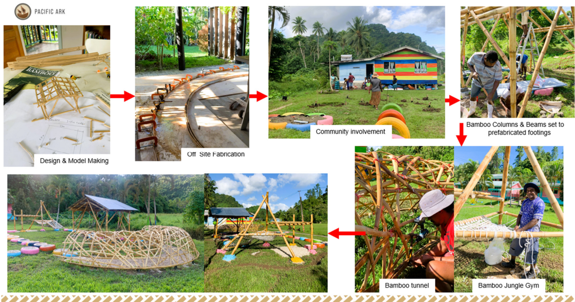
Figure 6-21: Urata Kindergarten bamboo playground: Step-by-step construction of demonstration bamboo build, from testing the bamboo's bending limits, framing to finished structures
