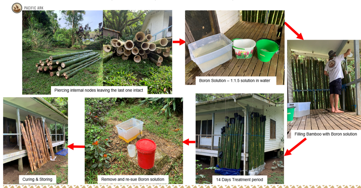
Figure 6-17: Vertical Soak Diffusion (VSD) setup for trials by Pacific Ark in Savusavu, Vanua Levu
