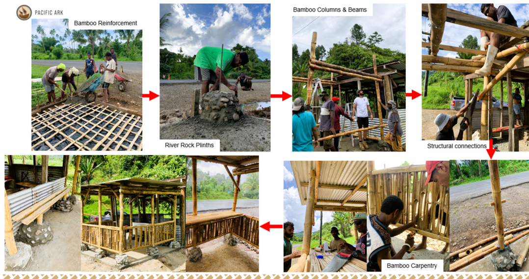
Figure 6-20: Da Roko Settlement Market Stall: Step-by-step construction of demonstration bamboo build, from framing to finished structure
