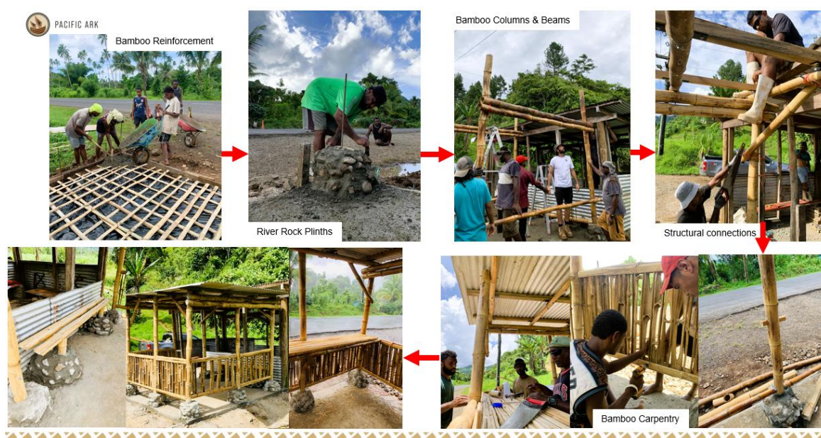
Figure 7-3: Da Roko Settlement Market Stall: Step-by-step construction of demonstration bamboo build, from framing to finished structure
