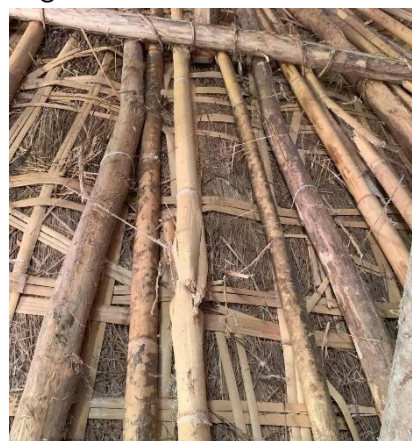
Figure 4-10: 15-Year-old Bure – sign of powder post Beetles and fungi
