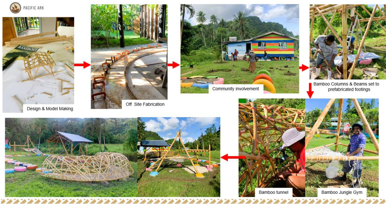
Figure 7-4: Urata Kindergarten bamboo playground: Step-by-step construction of demonstration bamboo build, from testing the bamboo's bending limits, framing to finished structures
