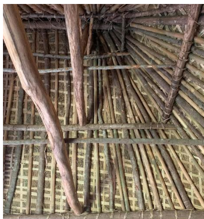
Figure 4-9: Use of bamboo for roof support trusses and thatching support bracing in bure
